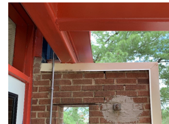
Photo #6 Brick Deterioration at Canopy Bearing
