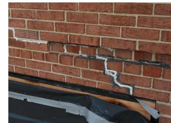
Photo #3 Typical Brick Crack & Repairs
