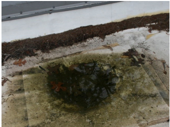
Photo #12 Clogged Roof Drain
