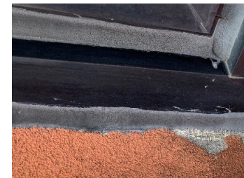
Photo #2 Typical EIFS Deterioration Bearing
