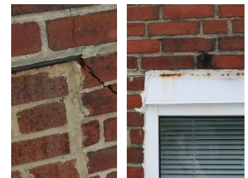
Photo #9, #10 Typical Brick Crack & Deterioration
