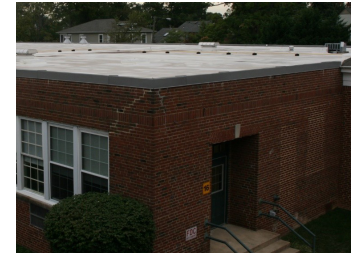
Photo #7 Typical Brick Deterioration & Repairs
