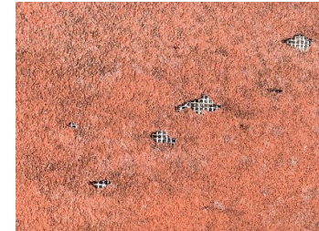
Photo #1 Typical EIFS Deterioration
