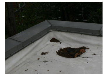
Photo #11 Clogged Roof Drain
